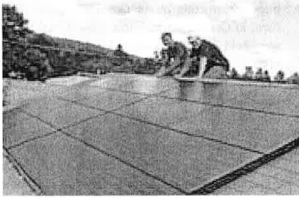
Solar panel installation, Cabot School, Cabot, Vermont.
