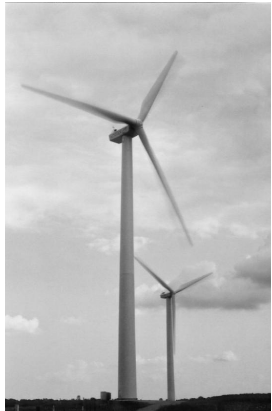
Green Mountain Wind Farm at Garrett, Pennsylvania
